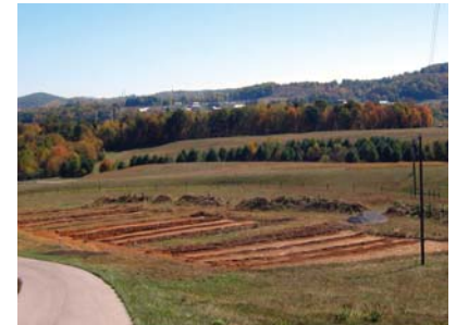
The research site after all soil treatments were installed (October 2007).
